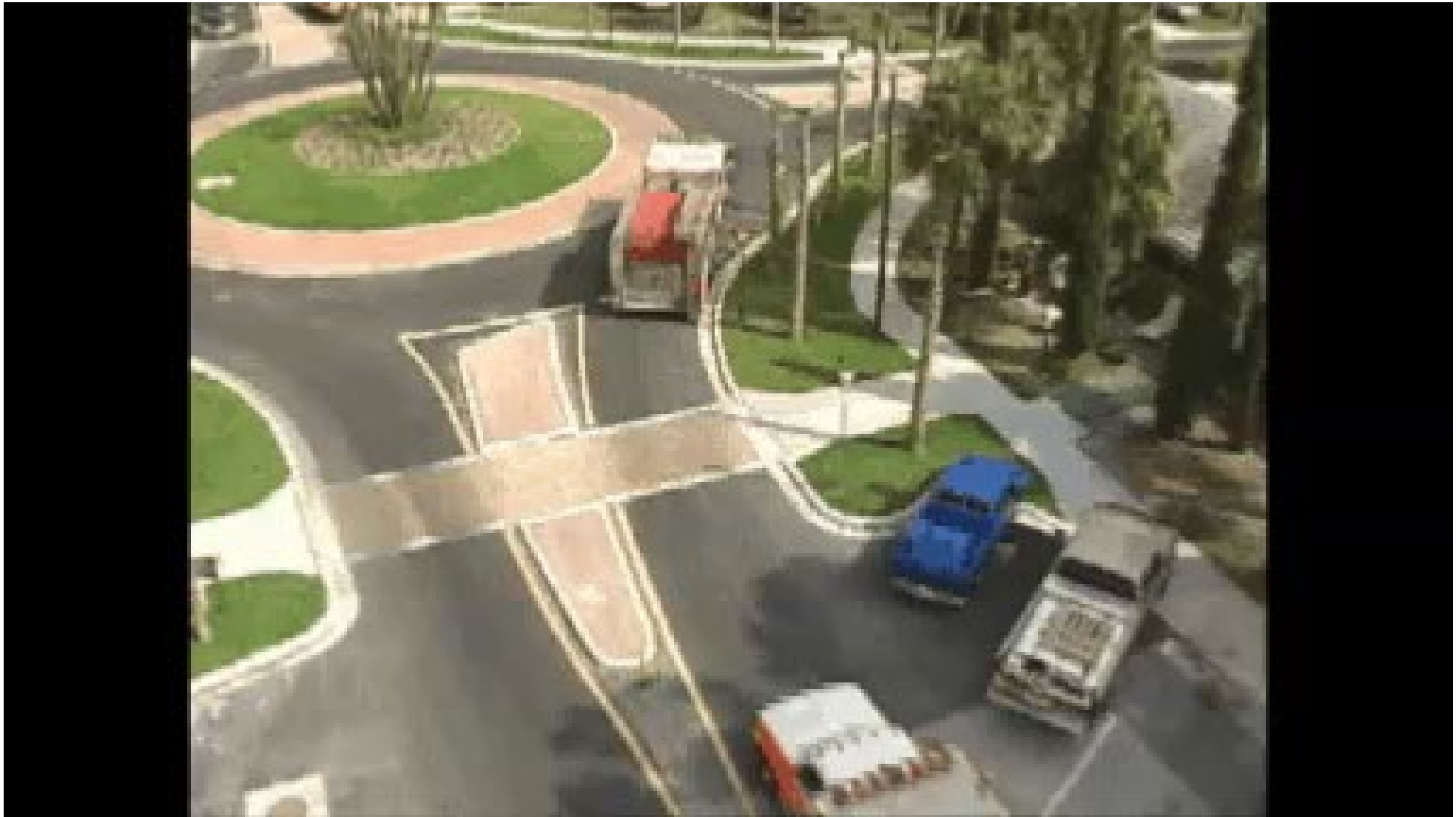
Emergency Vehicles Circulating Through Roundabout Courtesy of City of Clearwater, FL
