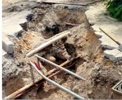
Open cut trenching
