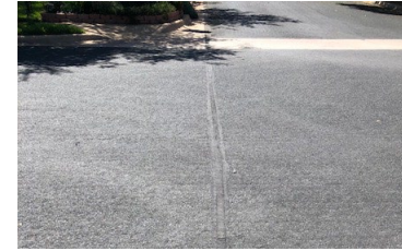
Example of a restored microtrench
