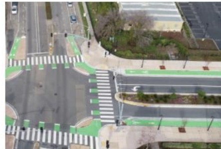
October 1, 2021 | Local Works | By Brian Hendershot
