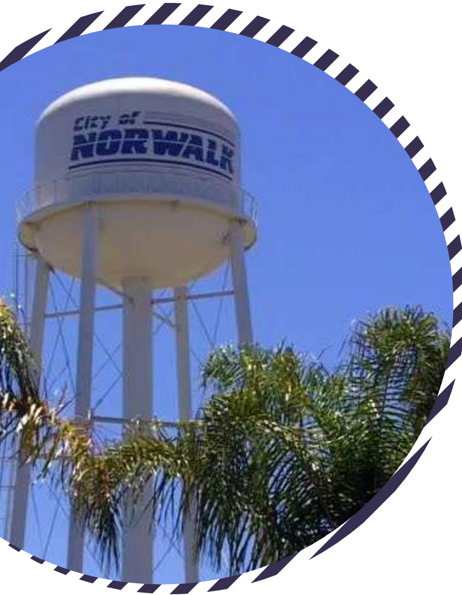
Figure 1: City of Norwalk Water Tower
