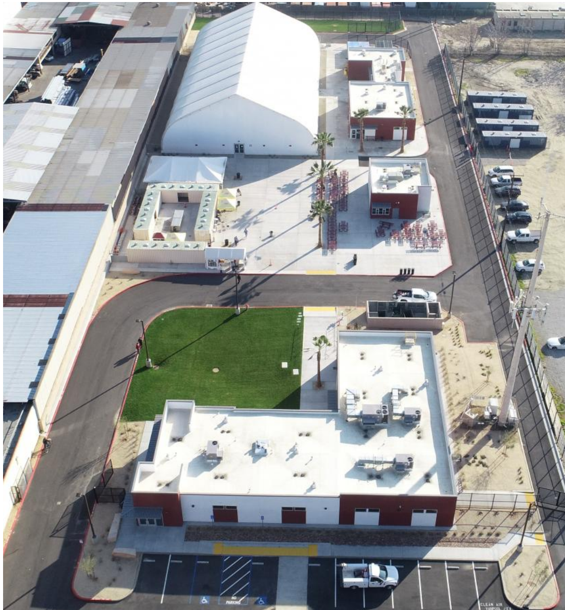
Pomona's Hope for Home, a 400 bed homeless shelter with wrap around services, expanded opportunities for Project Room Key locations, and tested the feasibility of community land trusts.
