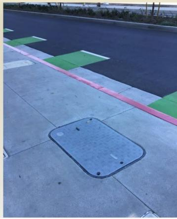
The system is a continuous loop so in order to maintain concentricity, vaults are placed in the ROW sidewalk or parkways to continue the run of conduits in the neighborhood.
