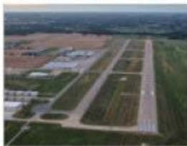
McKinney (Texas) Airport Expansion
