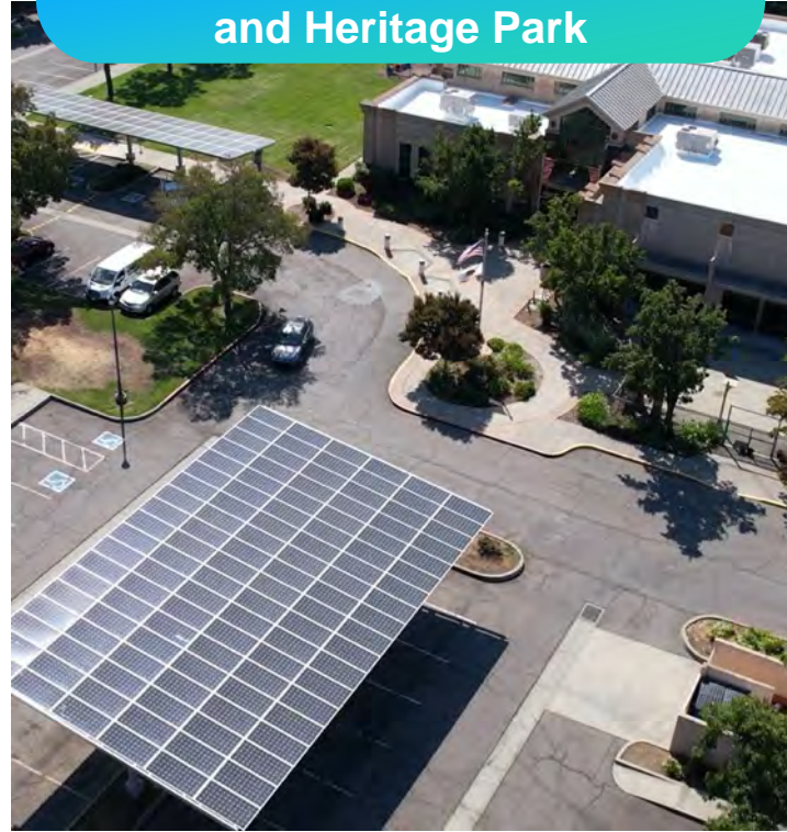
Parking Shade Canopies
