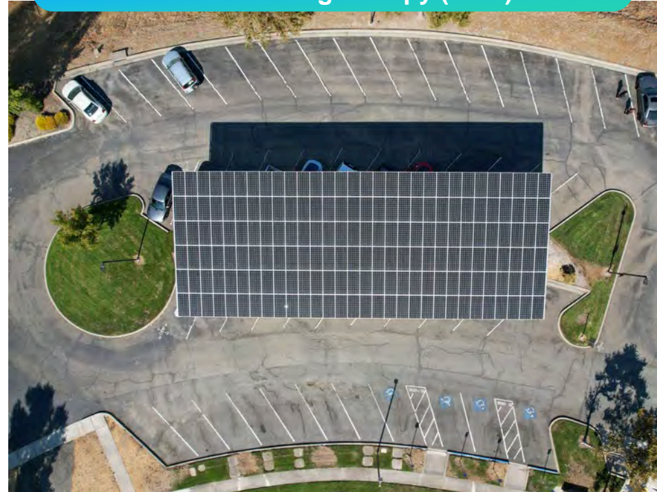
Visitor Parking Canopy (after)
